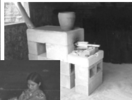
The new stoves (above) are constructed of cement and have a chimney to help keep smoke out of the home. The stoves are raised off the ground with an enclosed heat box that prevents children from getting burned.
