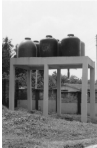
Water tanks are placed on concrete stands in Nigeria.
